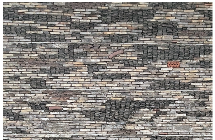
Wapan wall A façade of bricks and tiles rebuilt from the demolished community houses Photo: Yutaro Tomii
